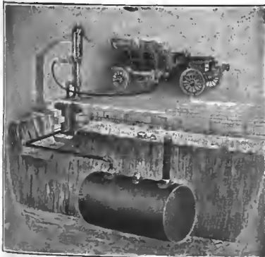
Cut 41—Long Distance Outfit. The Standard Garage Equipment for Gasolene Storage.
